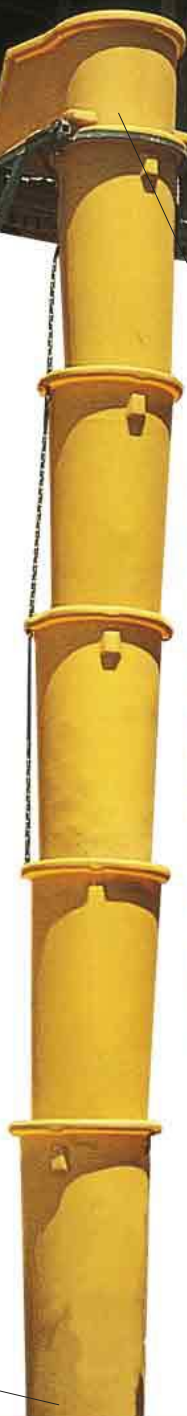
Top "cup" is attached to the building
