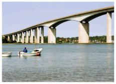
**Beam** A beam bridge is the most simple design. All the weight is placed directly on top. It is built to be stiff and not bend.
