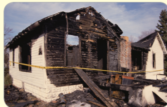
a burned house (The house is burned.)
