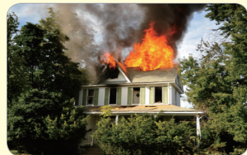
a burning house (The house is burning.)
