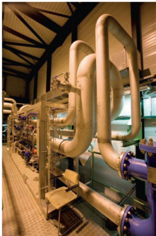
Above: One of the cryogenics plants supplying liquid helium to the Large Hadron Collider, the world's largest particle accelerator. The accelerator is a 27-kilometre ring in which protons are guided by superconducting magnets kept cool by 100 tonnes of liquid helium.
